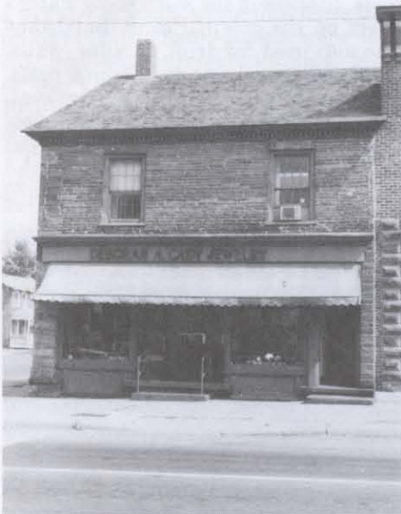
The first commercial use of Potsdam sandstone was in the construction of this building in 1821 at the corner of Elm and Market Streets, Potsdam, now a jewelry store. (Photo by Marian O'Keefe, SLCHA Archives)
